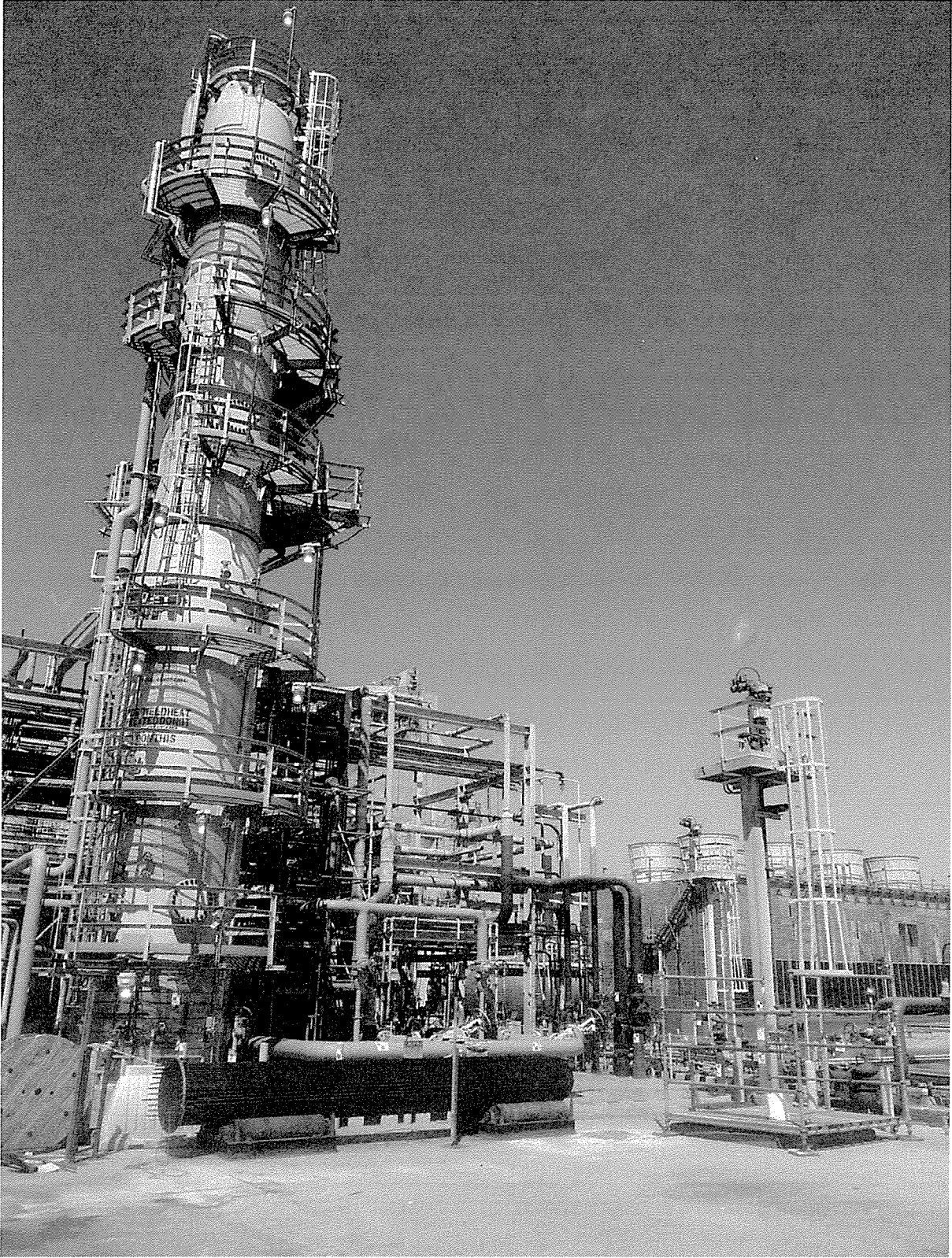
Picture of the Northeast Fire Monitor, Facing Northwest
